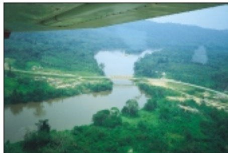
Bridges allow motorised traffic to formerly pristine areas.
